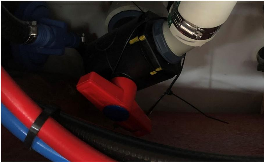
Valve closed, perpendicular to the line
